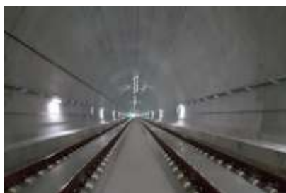
[Construction site of precast concrete track]
