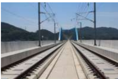
[Prefabricated concrete track]
