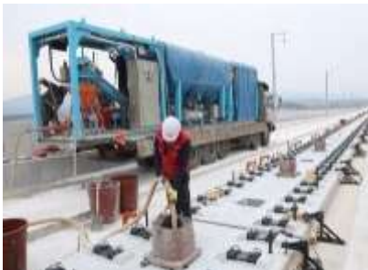
[View of prefabricated concrete track construction]
